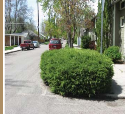
Example of a sidewalk and street obstruction
